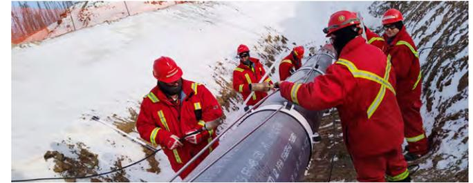
Fiber optic cables installation for the PLMS (pipeline leakage monitoring system) by Cameco
